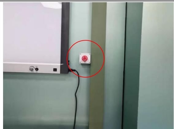
Pic10 机房内紧急停机按钮
